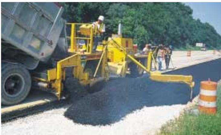
**Adjustable Wheelbase:** A bolt-in, removable frame section permits shortening the wheelbase/overall length 49" (1238 mm) to provide greater maneuverability on tight-quartered jobs.
