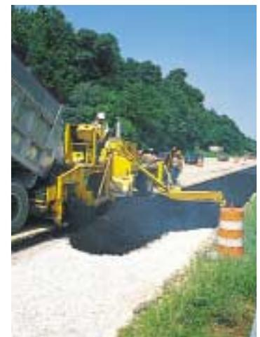
The conveyor will discharge material from either side of the machine. Discharge direction, left or right, is controlled with an electrical switch on the operator's console. Note that to accommodate opposite side discharge, it is necessary to transfer the strike-off assembly, hopper confining chutes, operator's console and seat to the opposite side of the machine. Unless otherwise specified, all RW-100A Road Wideners are shipped from the factory set-up for right side discharge.
