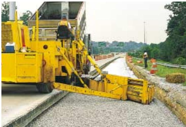
When shipping or traveling on the job, the strike-off can be swung flush with the side of the machine to limit overall width to 10'10" (3.30 m). A second strike-off assembly can be added to the opposite side of the machine to virtually eliminate the changeover time required in operations where frequent changes in right/left side material discharge are necessary.
