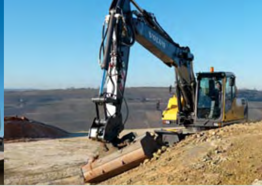
• Reach and power for dredging and ditching.
