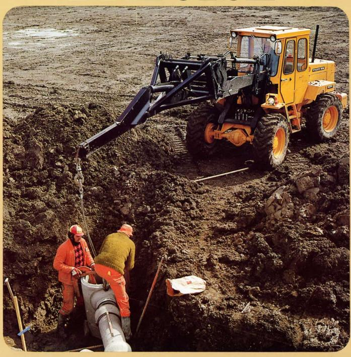
It's easy to work with the 4200 on difficult terrain. It has 4-wheel drive and low ground pressure. You can choose between two tilt speeds. The low speed is for precision work and difficult lifts. The loader unit works safely and surely, with high breakout force over its entire lifting range. The 4200 is a flexible machine, ideal for efficient working on a variety of construction site duties.
