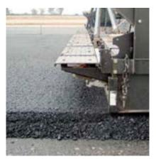
view of the low slump under the following roller, unevenness is reduced due to fewer roller passes. Outstanding evenness of the paved layer is therefore guaranteed.
